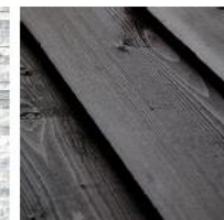
IMAGE 02: Painted timber cladding (Black)
